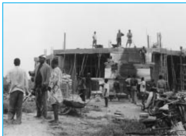
IMSP construction site
